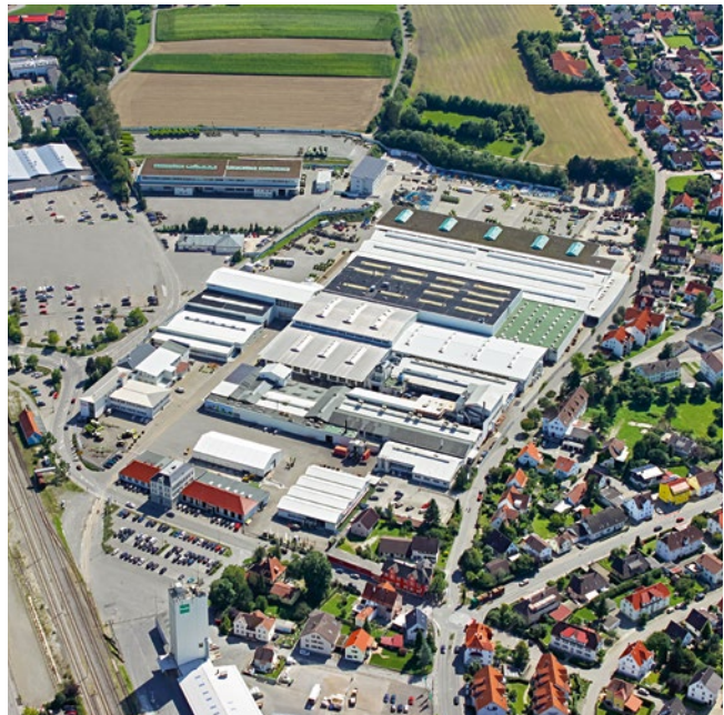
CLAAS Saugau GmbH in Germany is the company's forage harvesting center of excellence, with one of the most modern product development facilities in the world.
