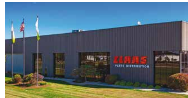
The CLAAS Parts Logistics Center in Columbus, Indiana, stocks more than 36,000 part numbers in a warehouse area of over 165,000 sq ft.
